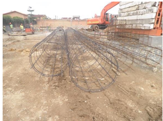
b) reinforcement of piles
