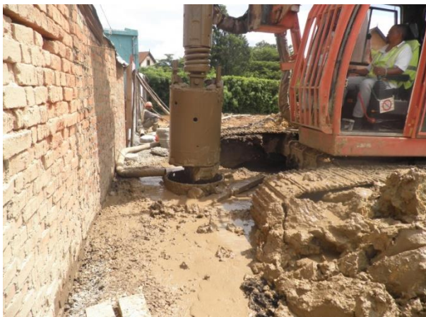
a) pile drilling
